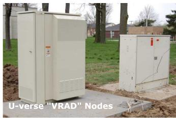
copper wire twisted pair to go from the box to your house. A purely fiber network would be faster, but by using their existing copper wire infrastructure AT&T is able to save a ton of cash by not having to dig up your neighborhood to run a new cable to your house. Still, with our residential gateway, or "RG" in U-Verse nerd parlance, reporting that it's capable of speeds up to 67 Mbps we can't really complain.
