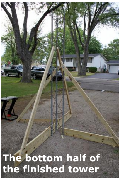
Bottom of the tower with all supports bolted in place
